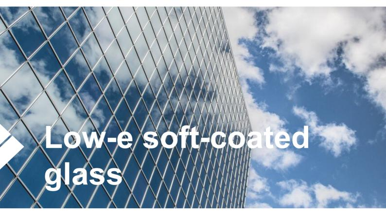
Low-e soft-coated glass is glass with coatings that enable a smooth penetration of solar radiation into the building and at the same time limit thermal leakage from the building to the outside world.
